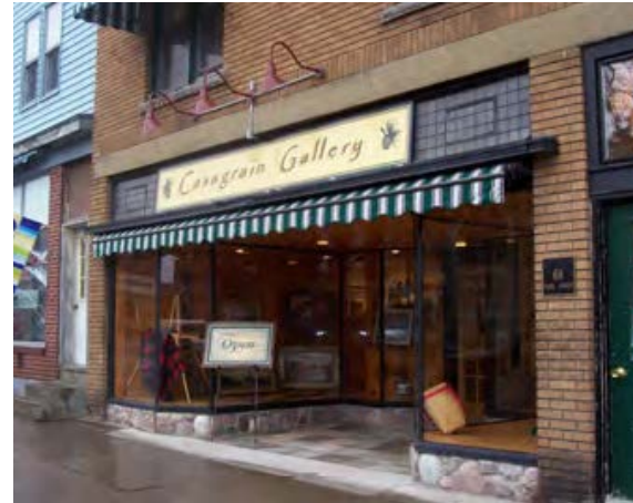
Transparent storefronts with awning and recessed entrance in Tupper Lake, NY. (Source: Tupper Lake Design Guidelines)
